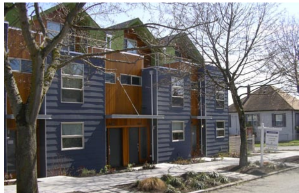
Composition of varied color, material and texture can create interesting townhouse façades as viewed from the street.
