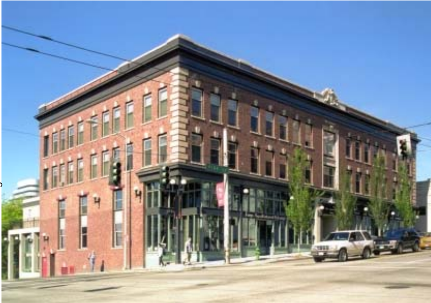
The shell of this existing brick apartment building was retained and reused. Behind and integrated with the old brick building is a new courtyard and five-story structure.
