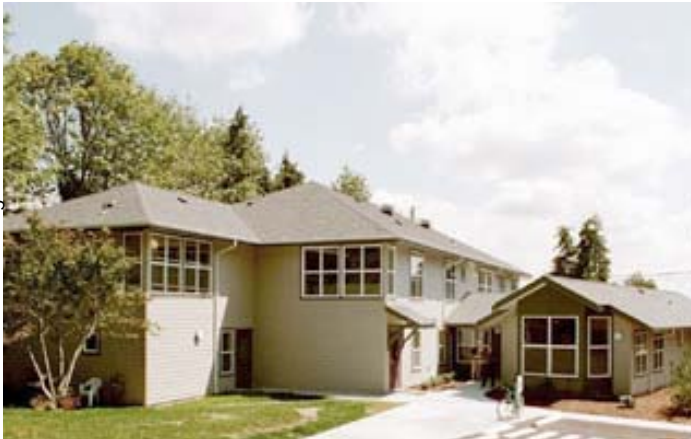
This affordable housing project used structural insulated building panels (SIPs).
