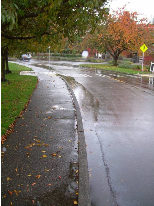
Figure D-1 North ADA ramp
