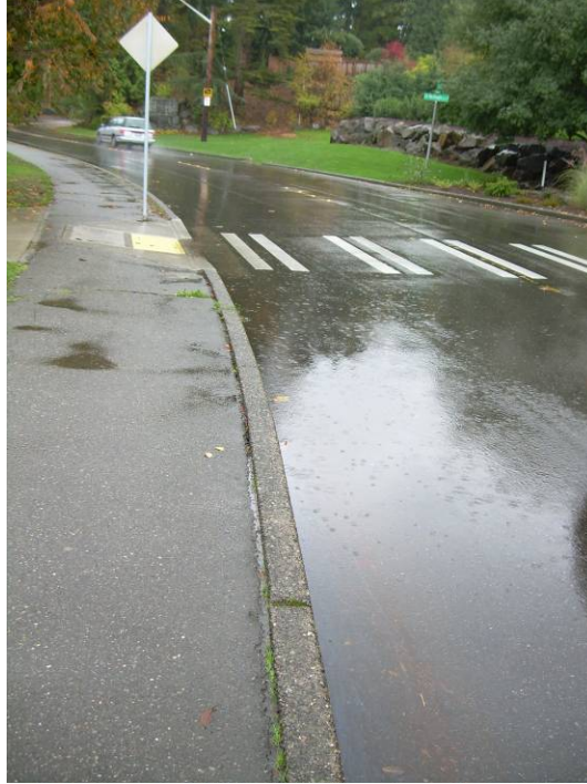
Figure D-2 South ADA ramp
