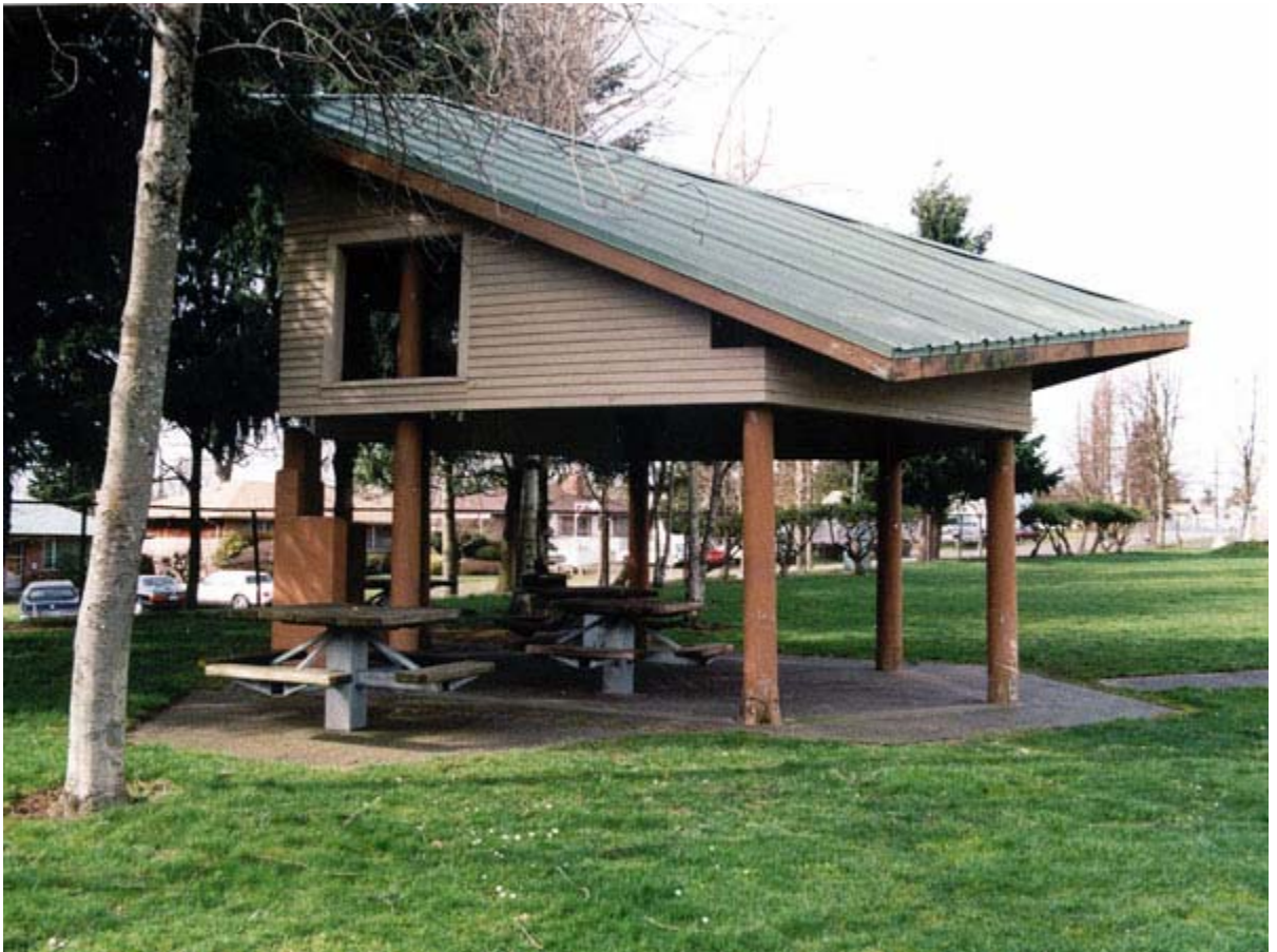
Benefit Playground picnic shelter
