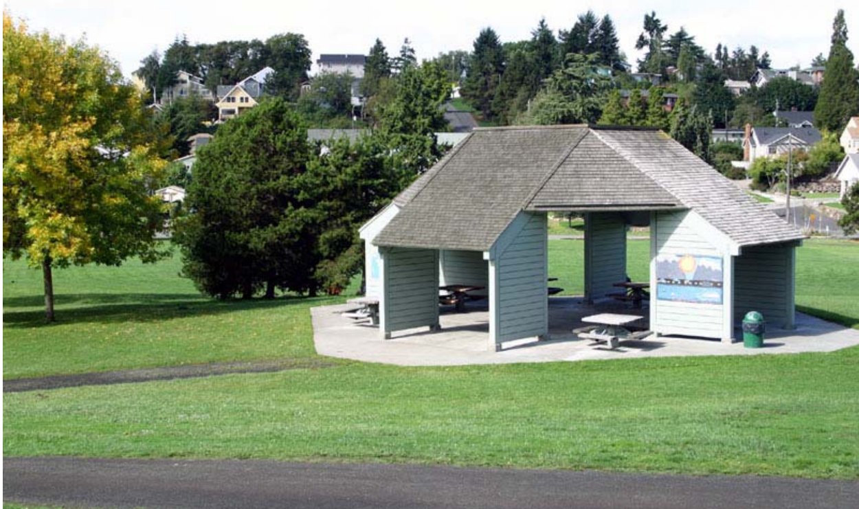
Genesee Park picnic shelter
