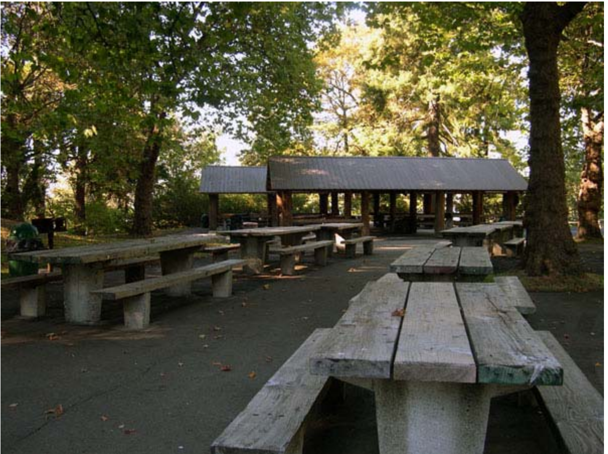
Seward Park Picnic Shelter 3 – more tables outside shelter
