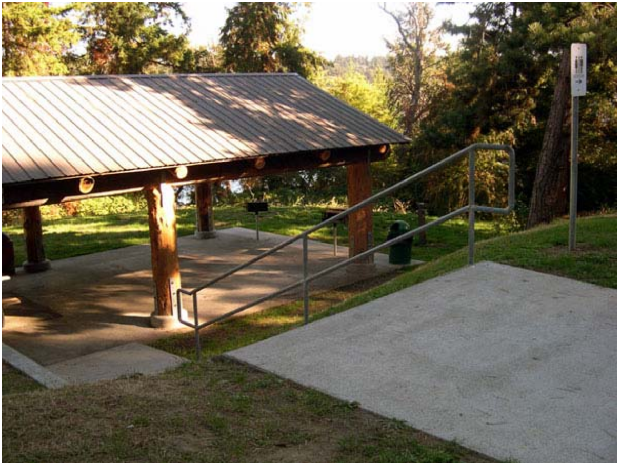
Seward Park Picnic Shelter 4 - Stairs to the shelter
