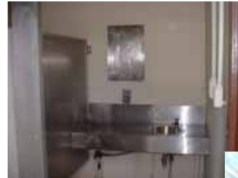
Bathroom upgrades will improve safety, ADA, aesthetics
